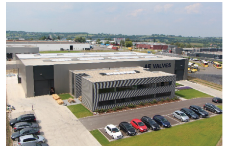
FIGURE 8 Emerson's AEV facility in Belgium
